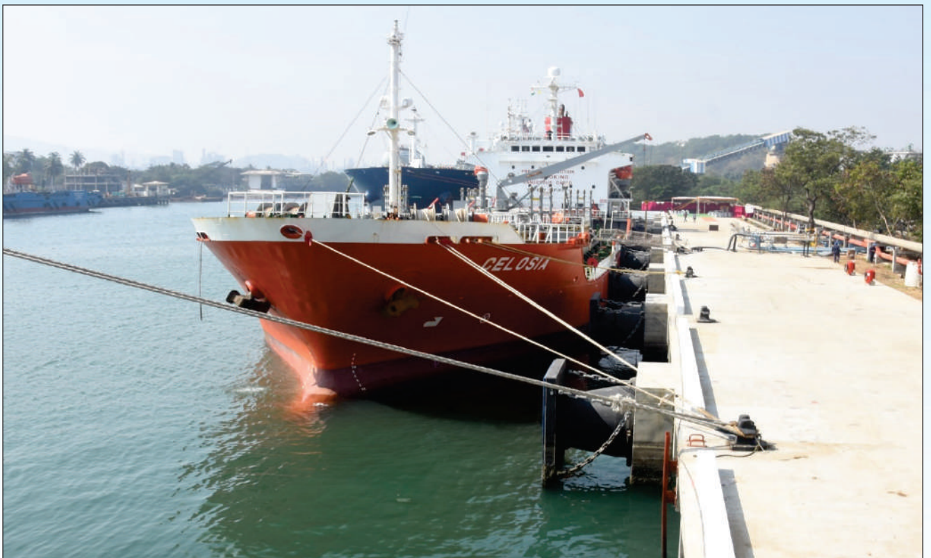
OR - III BERTH OVER VIEW
