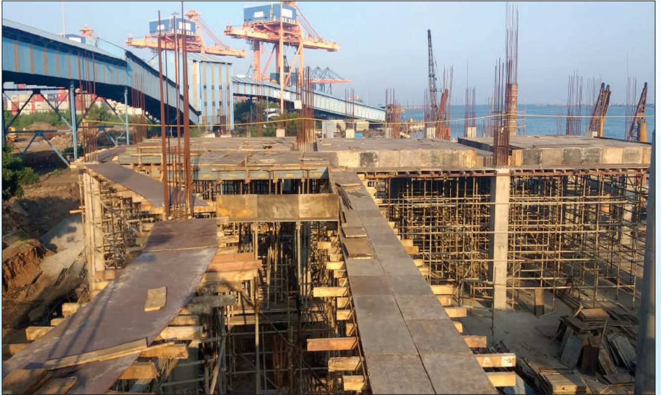
CRUISE TERMINAL BUILDING UNDER CONSTRUCTION PHASE
